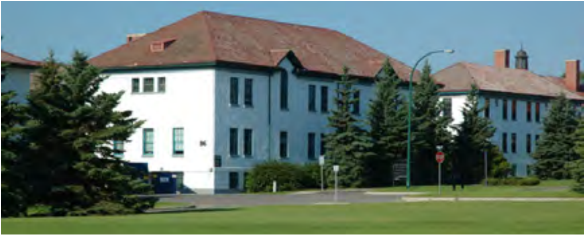
Historic Resources Buildings
