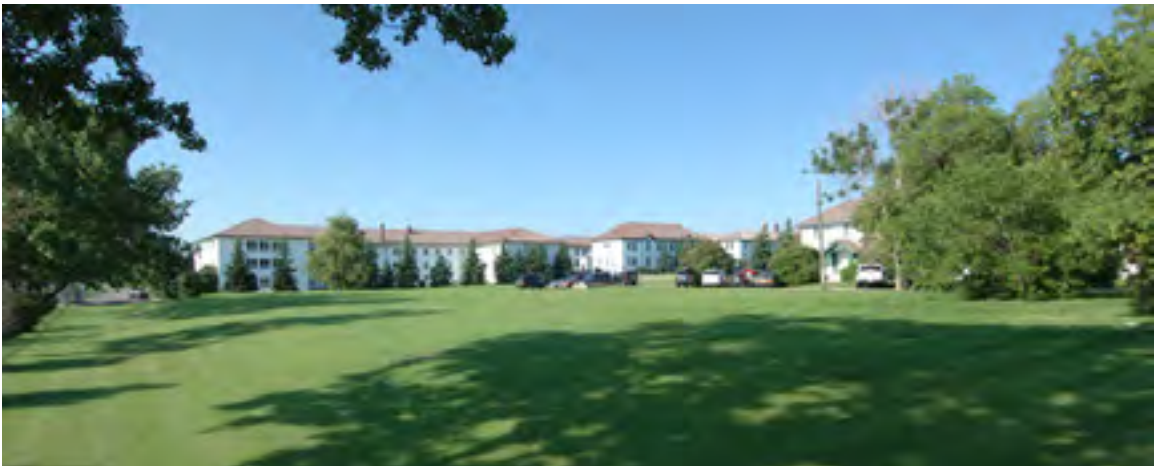
Existing Open Space
