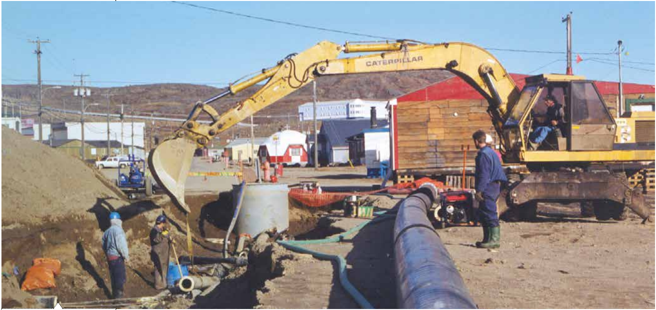
The piped water and sewer system utilizes insulated plastic pipe and steel manholes.
