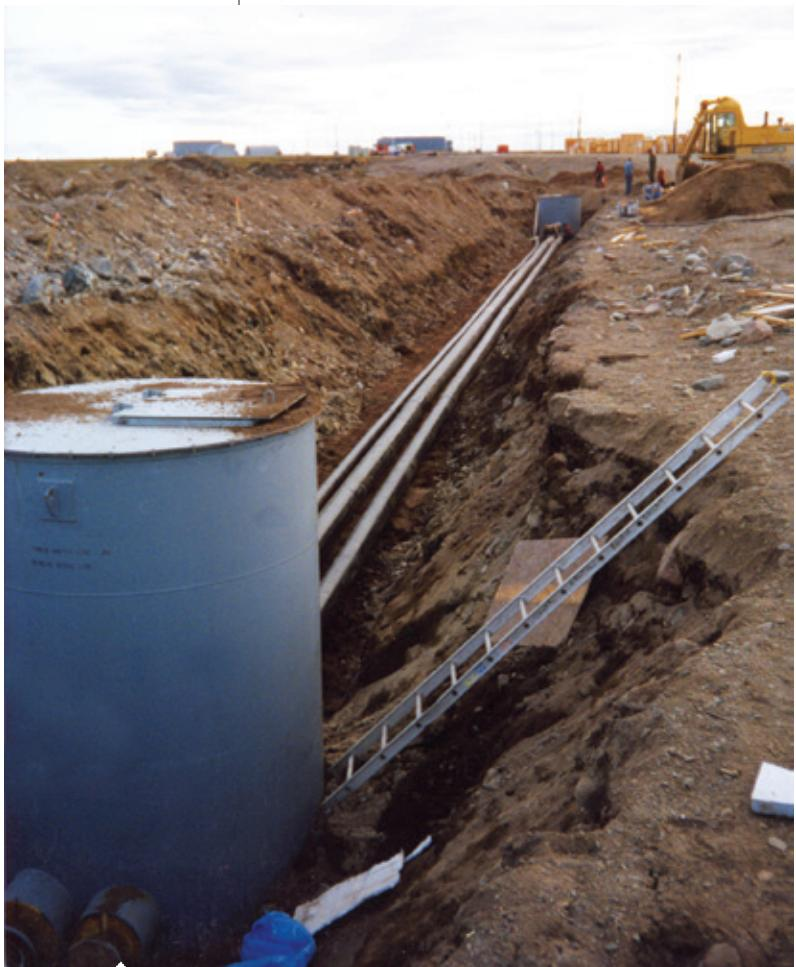
Buried, insulated High Density Polyurethane (HDPE) water and sewer lines between manholes in Rankin Inlet, Nunavut
